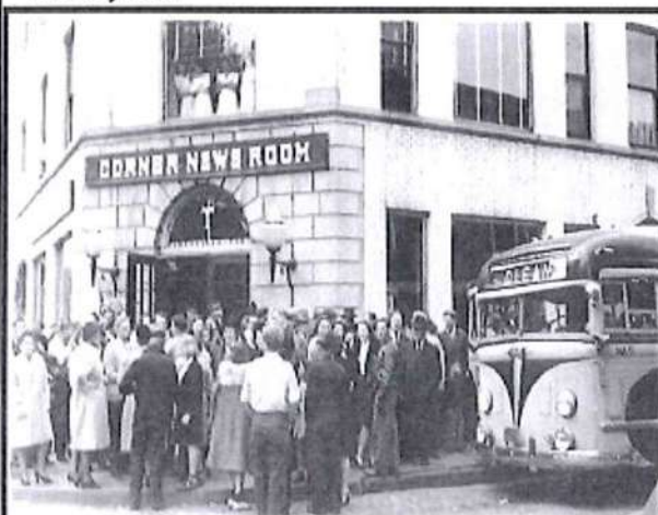
The Terminal Building, on the corner of South Avenue and Chautauqua Place, soon to be demolished. This photo was taken in 1941.
