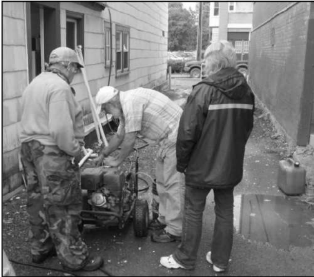
Dale adjusts the power washer while Tom and Molly look on – it took five hours to wash the building with ammonia and water.
