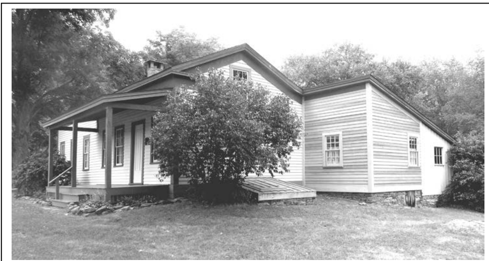
New siding on the farmhouse summer kitchen being repaired, summer of 2016.
