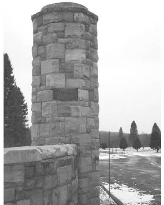
Gateway Tower to McKean Memorial Park Cemetery in Lafayette Township.
